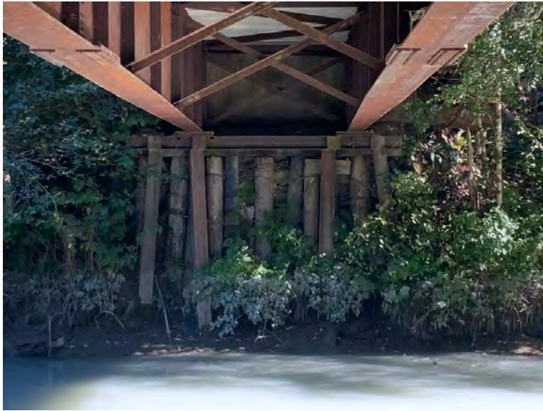
Left Bank Abutment when facing downstream
