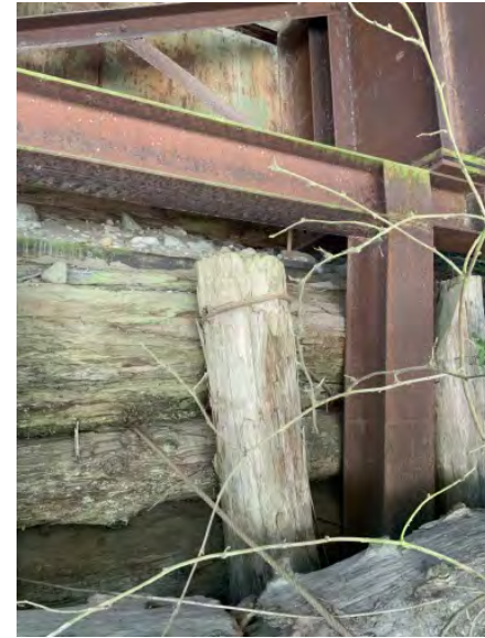
Right Bank Abutment when facing downstream
